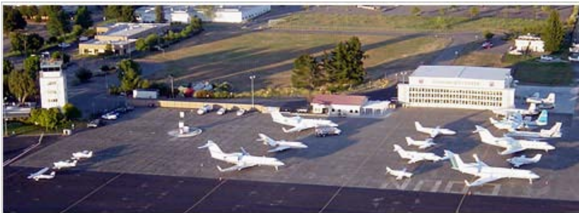
Fixed Base Operation
